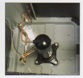
Carrier ships a spun copper filter dryer loose and it requires field installation
